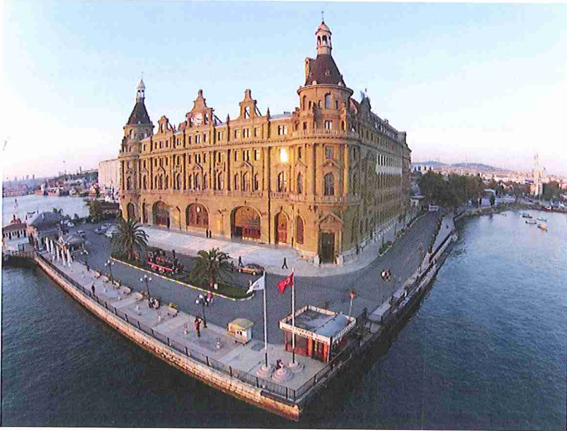
Haydarpaşa Train Station
